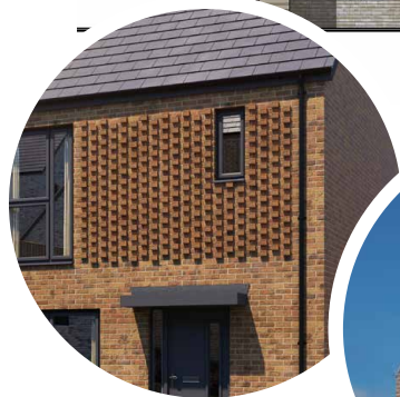
Brick Detailing & Slate Roofed
